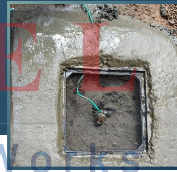
Earthing Pit Installation
